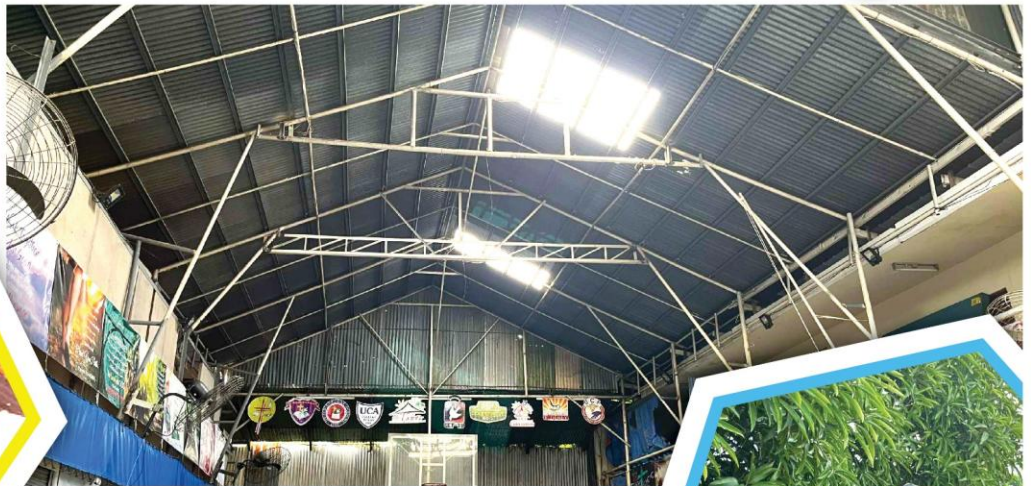
The newly repaired roof is now durable and has been restored for a better purpose, to guarantee students' safe learning environment.
