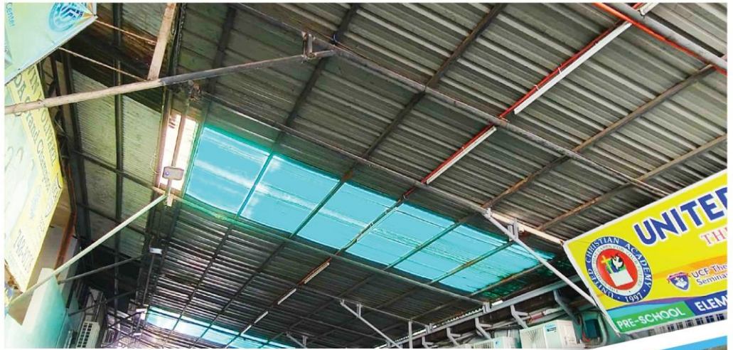
The holes in some parts of the roof were carefully repaired, and the metal supports were also painted. The steel beams were welded to ensure stronger support and stability.
